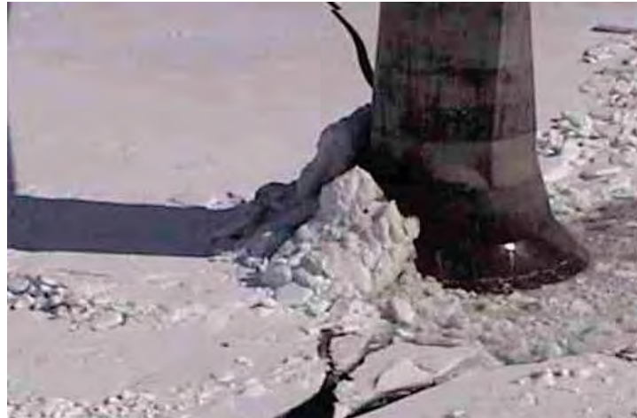
Figure 3.7: Upward Breaking Cone Fails the Ice, Minimizing its Load on the Foundation Structure 23
