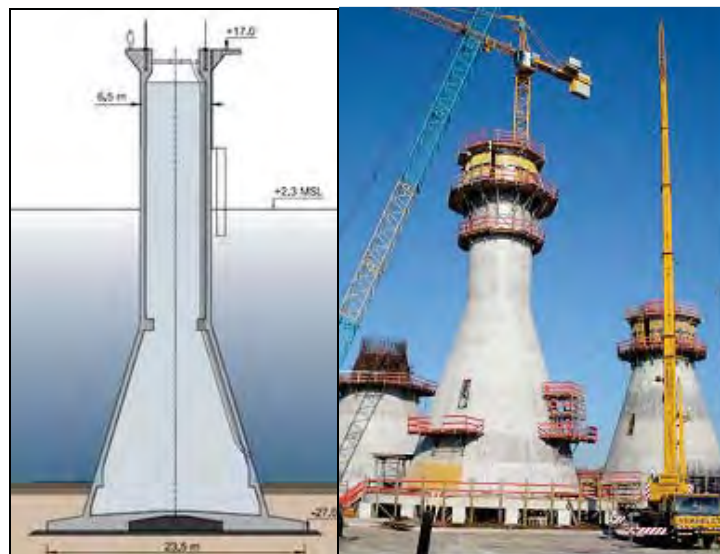
Figure 3.14: Gravity Base Foundation 35
