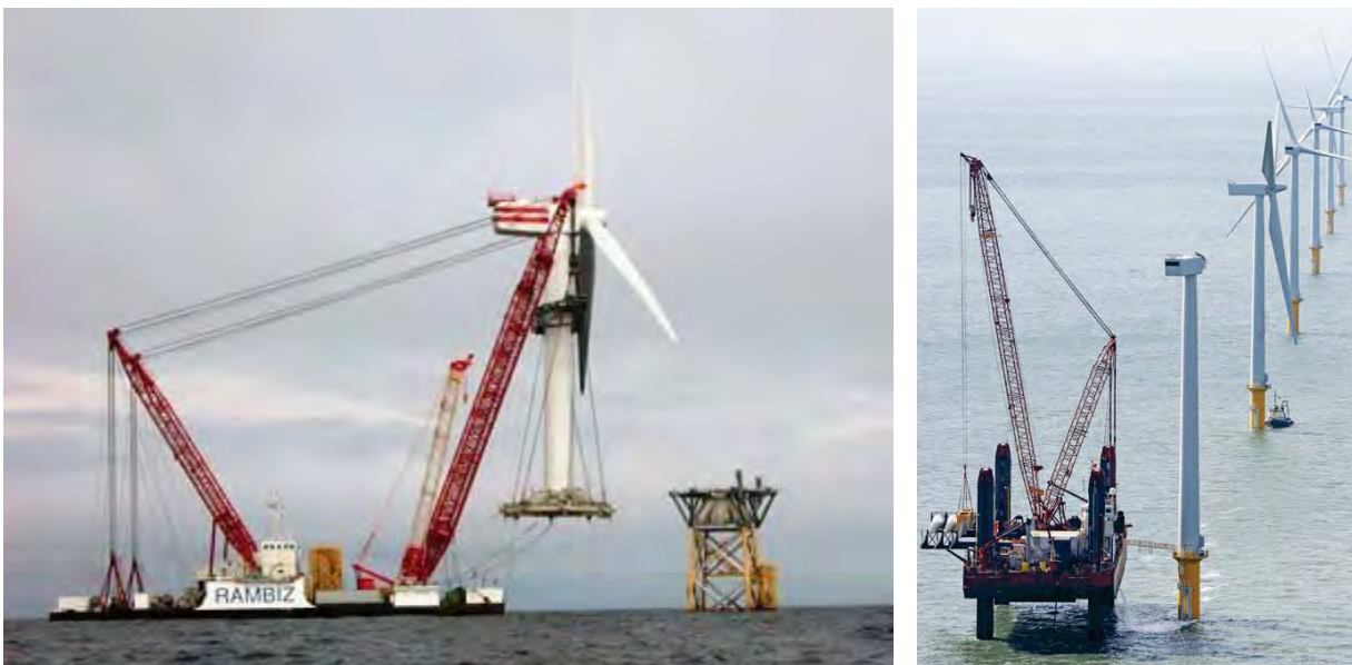
Figure 7.5: Heavy Construction Vessels Installing Wind Turbines 92,93
