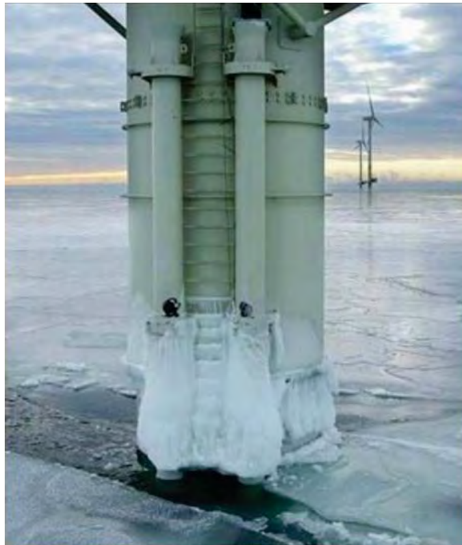
Figure 3.6: Turbine from Utgrunden Wind Project in Sweden Under Ice Pressure 22
