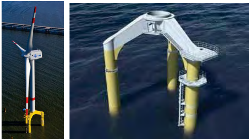
Figure 3.17: Tripile Foundation 40,41
